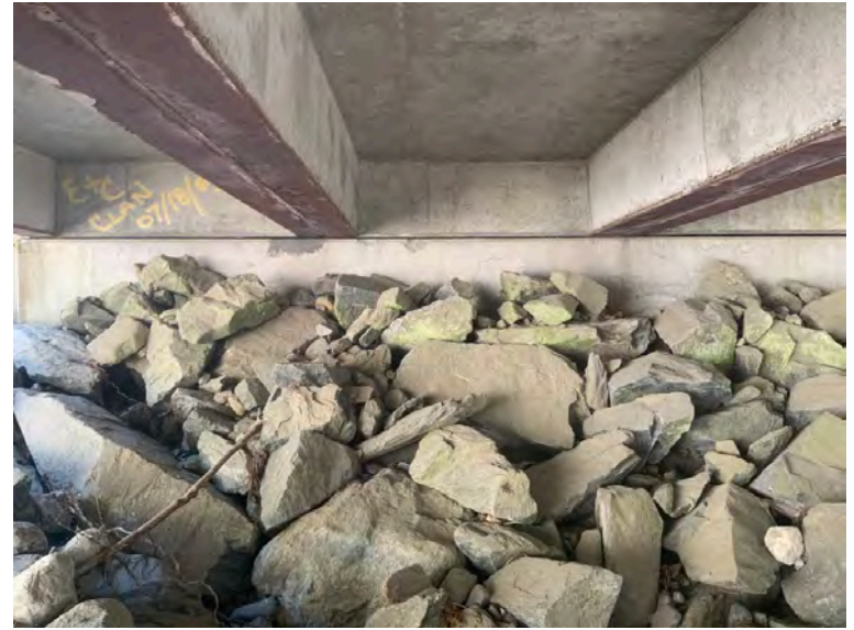
Left Bank Abutment when facing downstream
