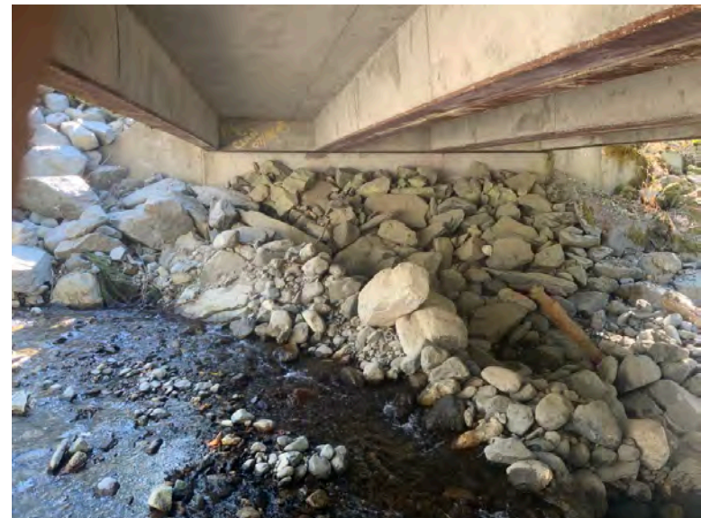
Left Bank Abutment when facing downstream
