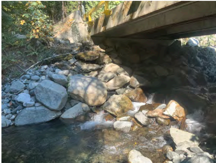
Right Bank Abutment when facing downstream
