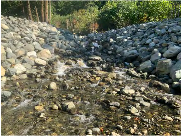
Upstream from Crossing
