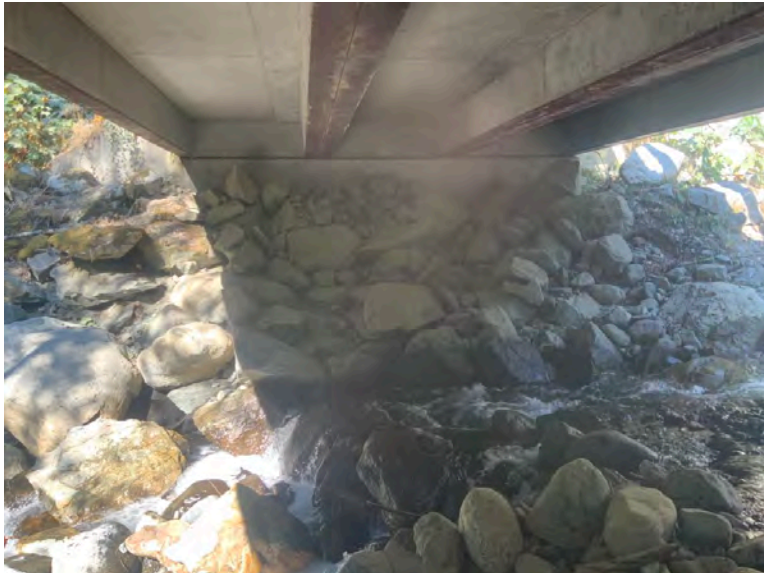
Right Bank Abutment when facing downstream
